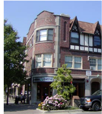
Northeast Corner of Elm Street and Chestnut Street
