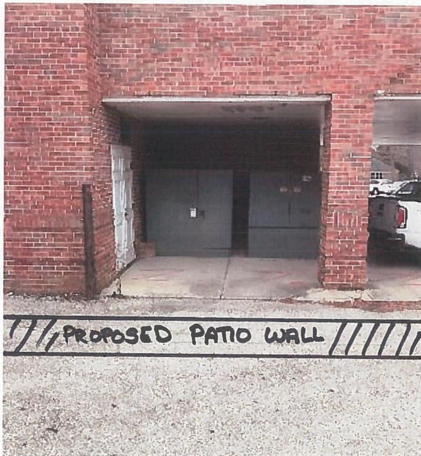
**Photo Of Transformer And Switchgear Beneath Building Overhang**
