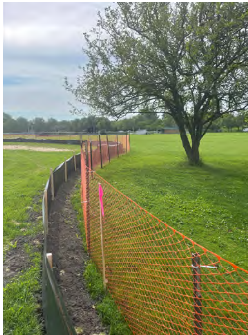
Orange construction fence and black silt fence ring the entire site.
