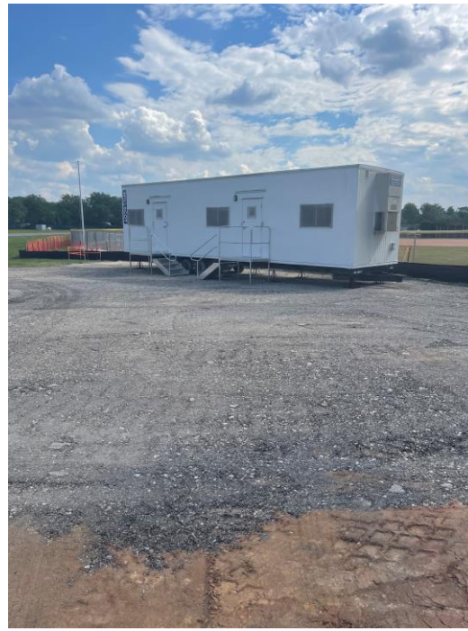
The jobsite trailer will be the hub for the Village, DiMeo, and Strand to make project decisions.
