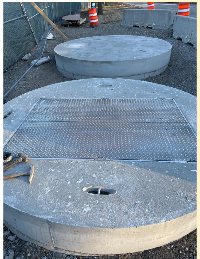
The Ash Street Pumping Station wet well received its hatch access
