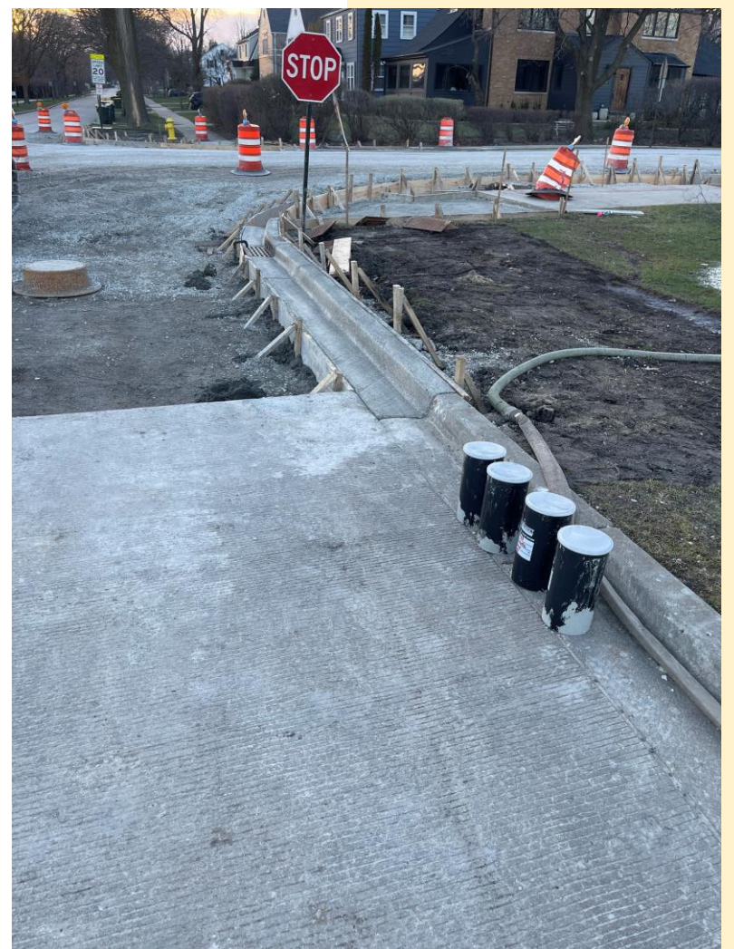
DiMeco completed restoration of the roadway at Hibbard and Oak
