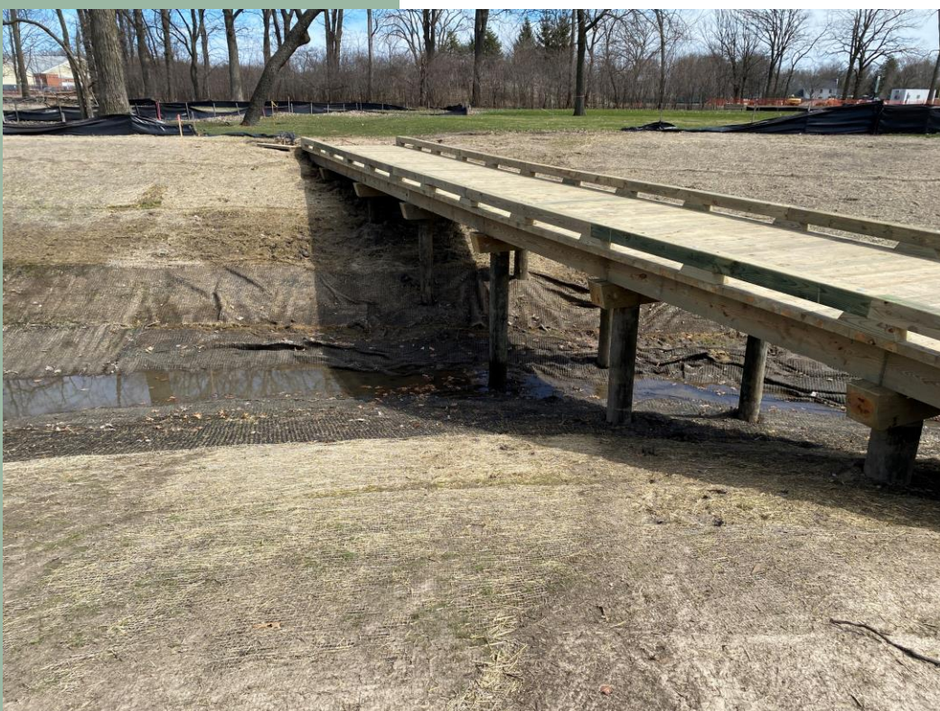
The final bridge on the Par 3 Course was installed this week
